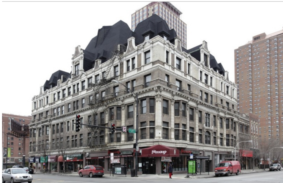
Cedar Street Cos. plans to buy the historic Bush Temple of Music building, built in 1901 and named a city landmark in 2001. Photo from CoStar Group Inc.
